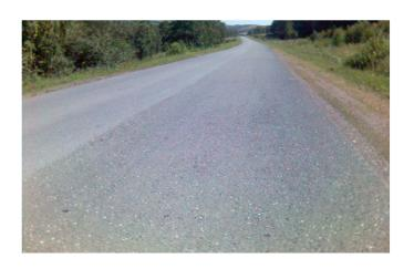
The section was built using unoxidized compounded road bitumen under the Technical Conditions of the Republic of Bashkortostan in June 1994.
